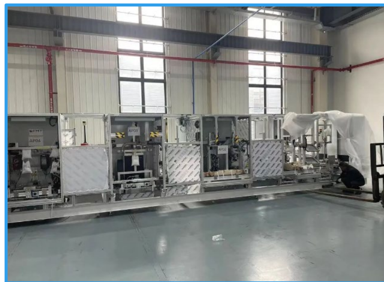
上海设备仓库内部照片 Interior photos of Shanghai Equipment Warehouse
